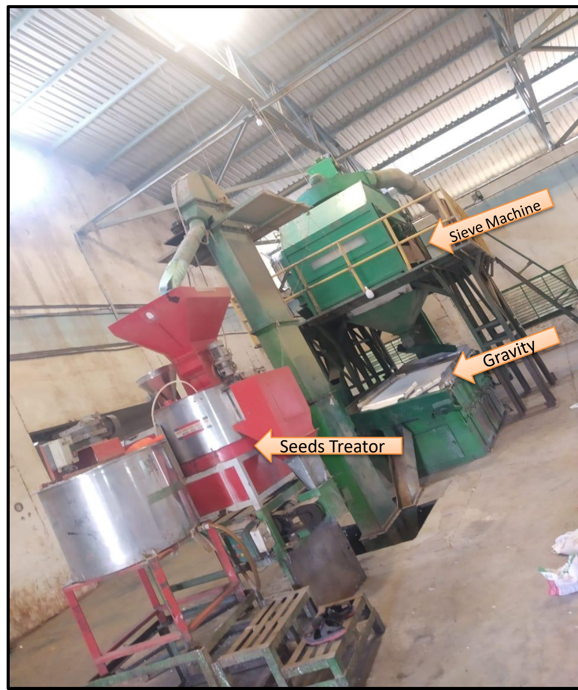
Seed Processing Plant
